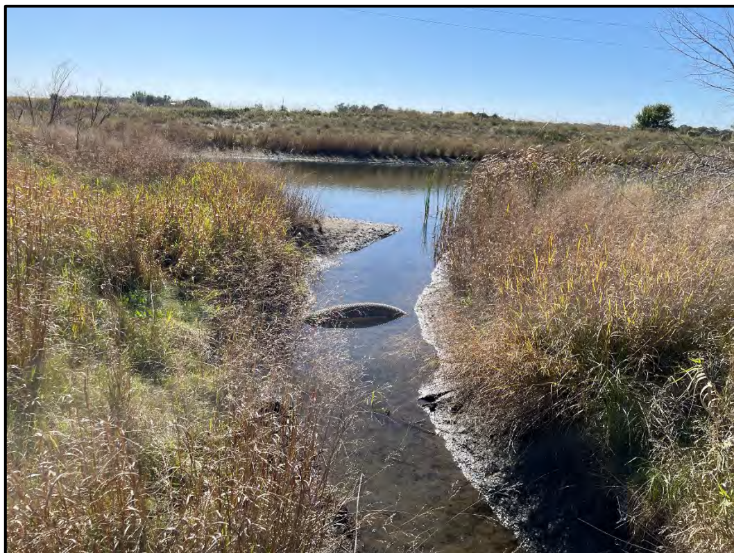
Excavated ditch on east side of the Substation, flowing south into the stormwater pond
